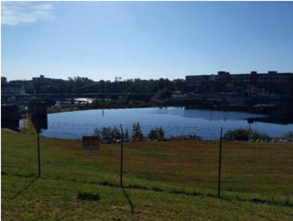
Source: I. Kiraly, Gomez and Sullivan Engineers, 10/03/2023
