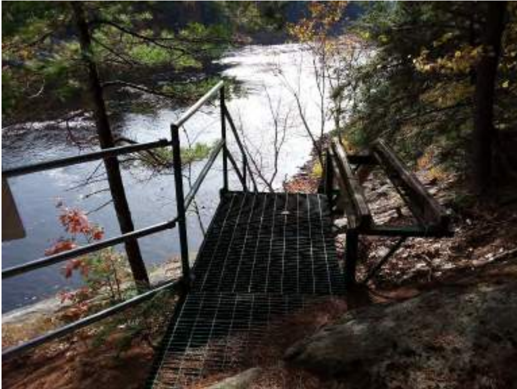
Figure 5.7.3.2-1: Pejepscot Dam Recreation Area, Portage Staircase
