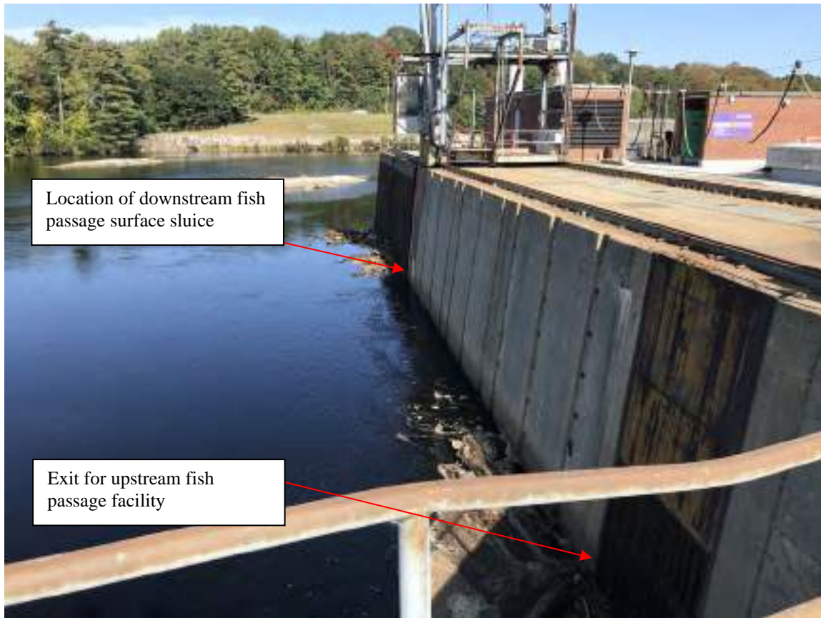
Photo 3-4: Project Turbine Intake Structure and Fishway Openings
