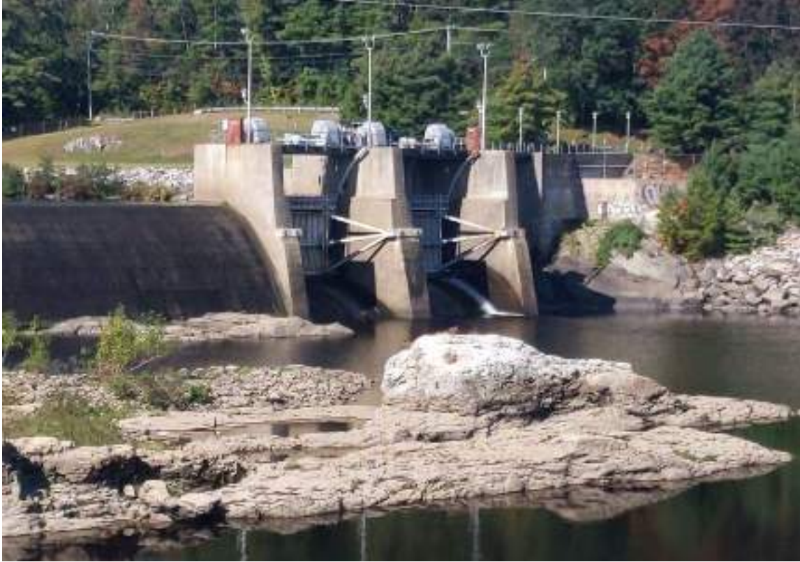
Photo 3-3: Project Tainter Gates and Emergency Spillway Sections
