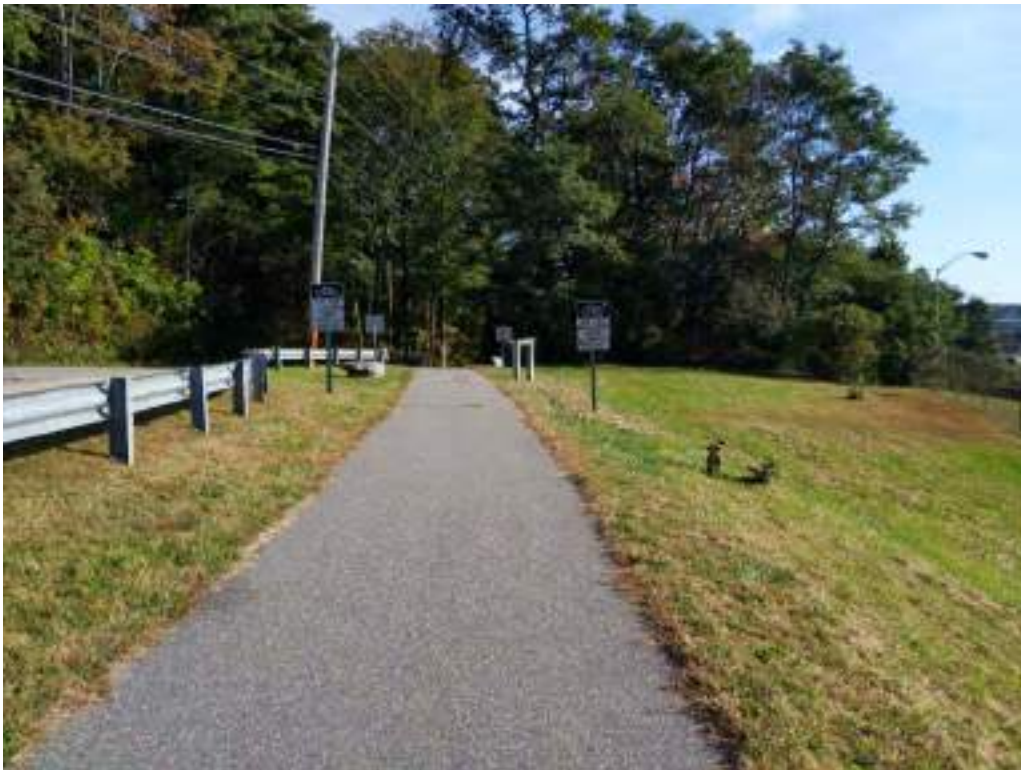
Source: I. Kiraly, Gomez and Sullivan Engineers, 10/03/2023
